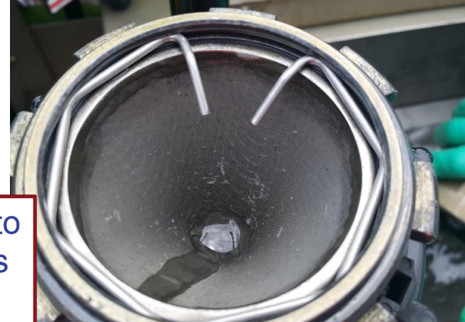
Hose-end strainer inspection/cleaning
